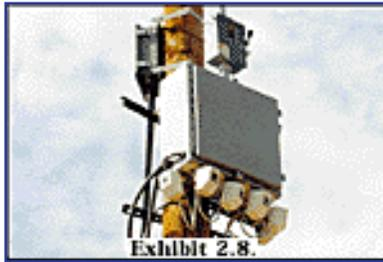
Short-distance, low-power RF wireless camera systems for video signal transmission are becoming more popular. (Wiring is still required for power.) A transmitter is required at the camera, as well as a receiver at the recording end. This will add an estimated \$1,000 or more to the price of the system for each distinct camera location (multiple cameras can be at one location, as in exhibit 2.8). In many cases,
