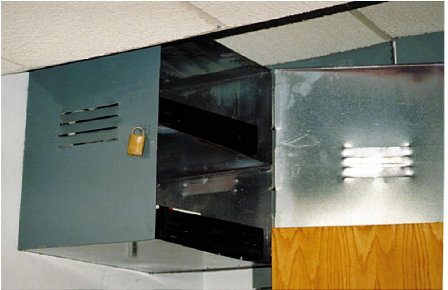
**Exhibit 2.15. This video recording equipment is protected by a simple locked and vented cabinet that resides within a locked room.**
