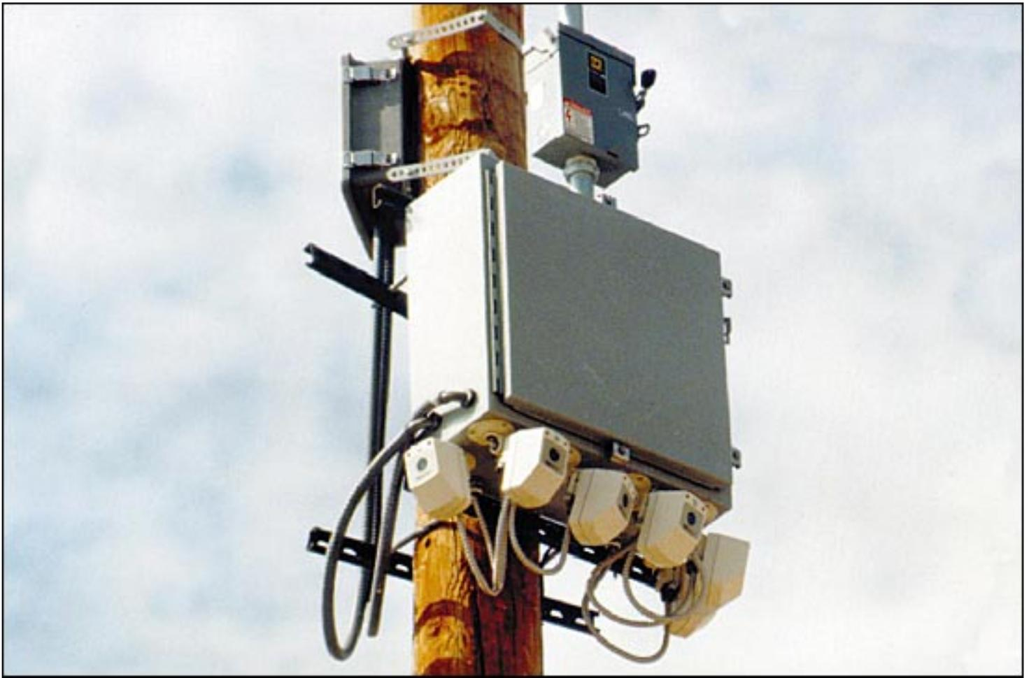
**Exhibit 2.8.** These bullet-resistant cameras on the light pole of a school parking lot were installed using wireless technology for data transmission. This configuration, which required line of sight between the transmitter and receiver, greatly reduced the expense and difficulty in running protected cabling back to the recording equipment. Note the protective shielding for the power cables that serve each camera.
