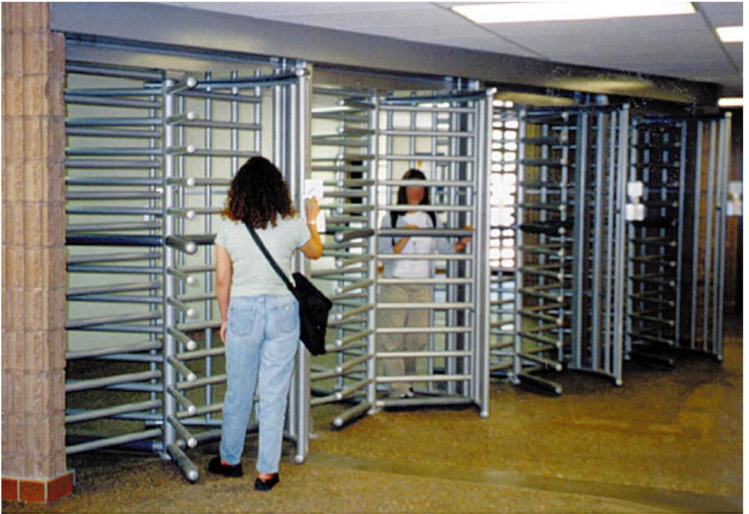
**Exhibit 4.3. These turnstiles operate when a valid ID card is scanned through the card-swipe device; this type of arrangement can prohibit more than one person from entering with one valid card.**
